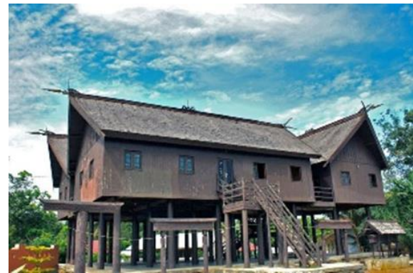
Fig 2_The traditional architecture of Indonesia, specifically the Minahasan (North Celebes) and Betang (Central Borneo) styles [8], [9]
